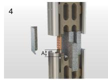
Support sheets are secured on the lower part of juncture area by stem bar. A min. 50-60 mm. The joint moulds are affixed on the support sheet by cleaning with a dry and clean piece of cloth.
